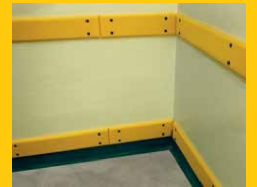
Wall buffers to prevent bumps and scrapes to surfaces.
