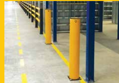
Bollards used to defend entranceway columns in storage facility.
